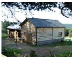
move them to the right place on the land. A separate specialist with a portable saw mill then came and cut the timber into planks for framing and cladding. The barn and garage were then constructed using part stone and blockwork and part timber framing with a slate roof. The finished buildings with local stone and timber grown on the land fit perfectly into the landscape.
